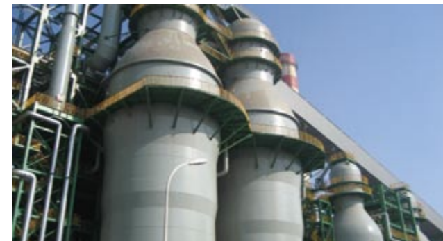
首钢京唐1号高炉热风炉 Hot blast stoves for Shougang Jingtang 1# blast furnace
