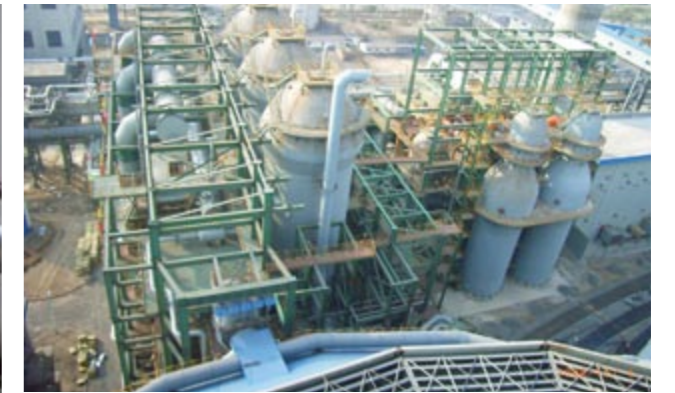
迁钢2号高炉热风炉 Hot blast stoves for Shougang Qiangang 2# blast furnace
